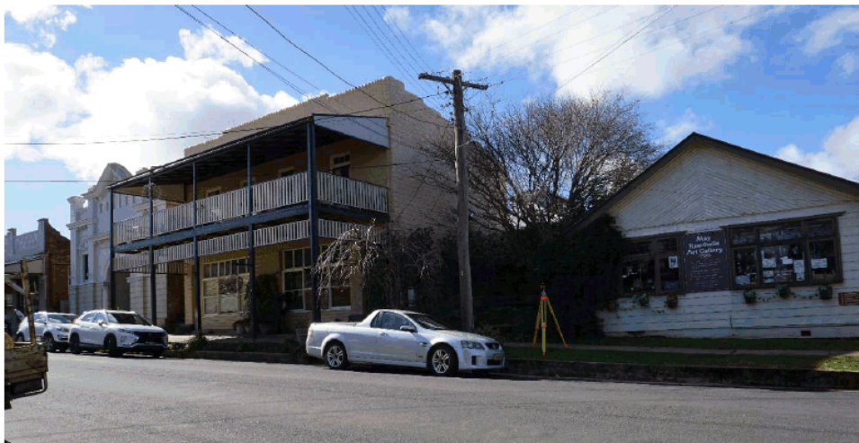
Looking North East at #8 Pym Street from opposite #10
