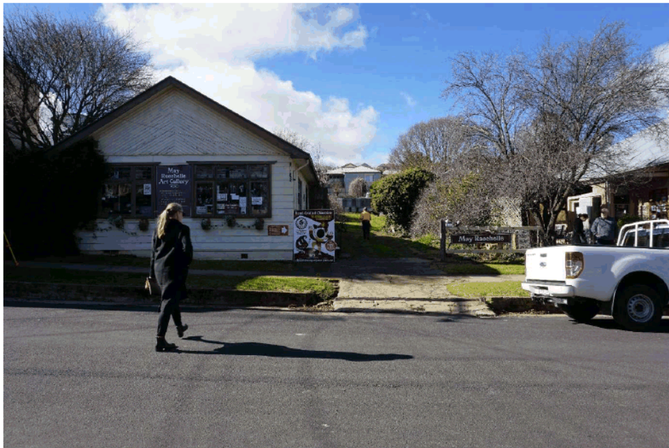
Looking East from Pym Street, adjacent #10. Old Mill Café on right (#12)
